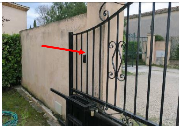
2 The key box is behind the gate
